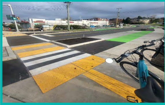
TACTILE WARNING AND DIRECTION SURFACE INDICATORS AT CROSSING LOCATIONS
