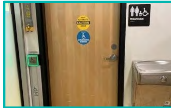
AUTOMATIC DOOR OPENER TO WASHROOM AT GORDON HEAD
